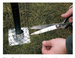
34. Continue to unroll the side netting all the way around the perimeter of your the door, unroll to about 30cm past the cage, keeping it as taught as possible, securing as step 31. When corners are encountered snip the bottom few cms in touch with the ground as shown to allow the net to neatly fold.
