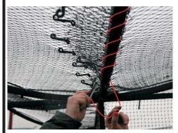
46. With the whipping needle loaded with twine, tie one end of the twine through the slot in the appropriate connector plate. Then feed the needle around the horizontal bar to neatly tie in the nets as shown. Finally tie off the twine through a slot in the opposing connector plate. When you are completely happy with the result, remove all of the net clips (ref. 26) and trim off any untidy net edges with scissors.
