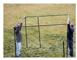
16. Locate the square unit into the tops of the uprights and the door support upright as shown above.
