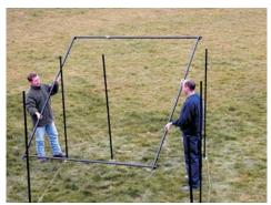
14. Locate the door support upright(s) (ref. 4) such that the gap between it and the upright that the door will hinge from is 770mm (between inside faces).
