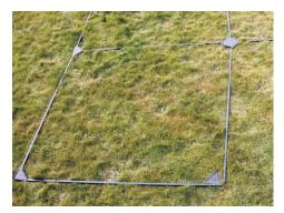
After reading the introduction, lay out on the ground in the desired arrangement of the final cage all 2.5m horizontal support bars (ref. 14), all connector plates (ref. 18,19, & 20) and all three, four & fve way connectors (ref. 15,16, & 17).
