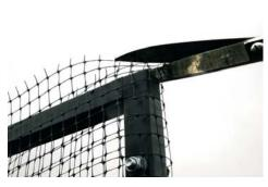
Trim the net level with the top of the door as shown. Any side net sticking ties (ref. 27) as shown. up above the top edge of the 2.5m horizontal bars around the perimeter of the cage can also be trimmed.
