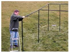
17. Locate any other complete square horizontal bar units as in step 15 as applicable. Then add all other horizontal bars one at a time until all horizontals are in place. Make sure that all threaded holes on the horizontals are facing upwards.
