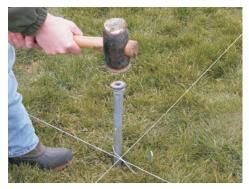
10. With the aid of a mallet and a stake, carefully create appropriately sized holes in the ground about 32.5cm deep the foot plates (ref.13) as shown. The to receive the uprights (ref. 4). The uprights can be concreted if required but do not set until the steel framework is fully assembled and levelled. (You may find a hole former (ARC-021) useful for making the holes.)
