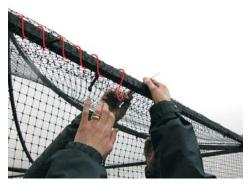
46. Tie in the sides of the roof net(s) to the horizontal bars and side net by using the twine and whipping needle as shown above again trimming where necessary. Net clips (ref. 26) can be used to aid in this process.
