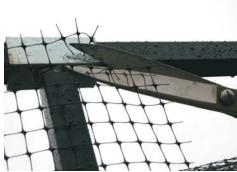
32. To fix the 2m wide side netting, start by cutting as shown to allow the net to wrap around the door support upright. This will allow the top edge of the net to run along the top edge of the horizontal support bars.
