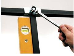
22. Check that the door support upright (ref. 4) is vertical and then tighten the bolt with a 13mm spanner.
