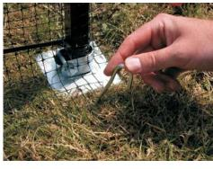
47. Walk around the perimeter of your cage and insert ground pegs (ref. 25) (as shown above) approximately three per meter to secure the bottom on the side net. Check that the top edge of the side net lines up with the top edge of the horizontal bars, trimming where necessary.
