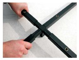
3. Using the correct connector (ref. 15,16 & 17) for the joint in guestion, connect the 2.5m horizontal bars (ref. 14) together to form a framework of bars which represents the roof of your cage (in plan form) on the ground. The soft mallet may be needed to help slide the bars home.
