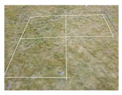
9. Your site should be marked out in the manner shown above. If your site slopes, level the strings with the aid of a spirit level. Position the door on the lowest side of the cage if possible to ensure that all of the uprights (ref. 4) can enter the ground at least the required distance of 32.5cm.
