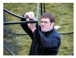
28. Bolt (ref. 22 & 23) the curved roof 29. Tighten the bolts using a 17mm supports (ref. 24) onto the connector spanner. plates (ref. 18,19 & 20).
