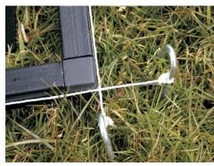
5. Using string tied to ground pegs (ref. 25), mark out the plan of the cage on the ground as shown above. Where ever the strings cross, this accurately marks the intended position of an all is square as described in step 4. upright (ref. 4).
