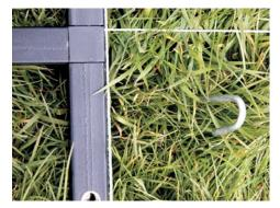
7. When more than two horizontal bars come together, it is essential to mark which side of the string the uprights will be located. Ground pegs (ref. 25) can be used for this.
