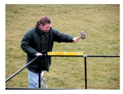
21. On side(s) of the cage that door(s) to the top face of the horizontal bar. With a soft mallet, tap the uprights into the ground until this measurement is 2 meters. Check that the horizontal bar is level and that the previously assembled door frame will fit under the bar.
