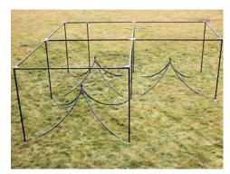
25. Assemble as many roof units as required for the constructed framework and place inside the cage as shown. Then place a ftted roof net over each roof unit.
