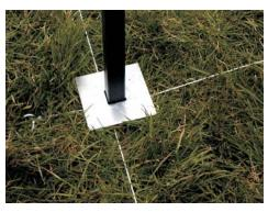
11. Place the uprights (ref.4) into the holes and at the same time slide on uprights should be pushed into the ground approximately 30cm at this point.
