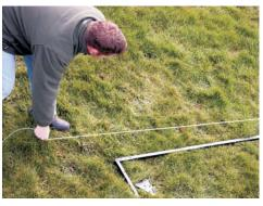
Ensure that the marking string is pulled tight and accurately follows the framework of horizontal bars which act as a template. Check once more that
