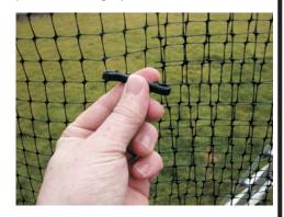
36. Fold the side net around the catch side of the door and hold securely with several equally spaced net clips (ref.26). A small cut can be made in the net to allow the catch to protrude cleanly.
