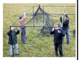
27. With the aid of at least three people, lift the roof unit(s) into place as shown. Have the washers and bolts to hand when you lift the roof unit(s).
